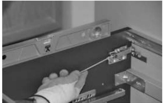
d\_ The leveling on the depth of the furniture is made turning the lower screw, as shown.
