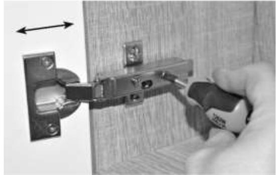
c\_ DEPTH: This regulation is made by the most internal screw.
