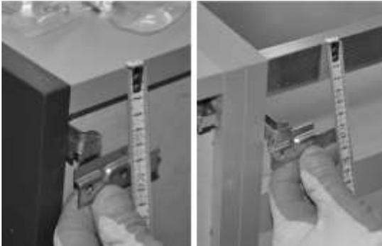
a\_ For the positioning of the brackets, consider that the height for a neutral unit (fig. 1) is different from a washbasin unit (fig. 2).
