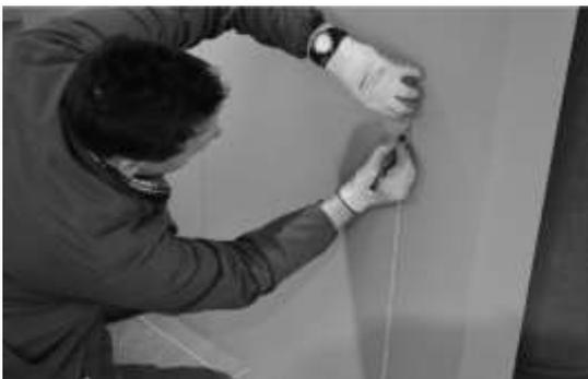
c\_ Detected all the necessary quotes, proceed to the mark points on the wall for drilling and insertion of the dowels (\*).
