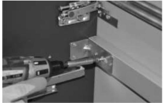
e\_ Once fixed the furniture with hangers, we will proceed to secure fixing with supplied screws and dowels on the posterior chain of the cabinet.
