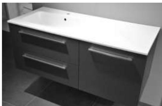
e\_ Once verified the perfect condition of the cabinet and the installation, proceed with the fixing of the top being careful to use neutral silicone.
