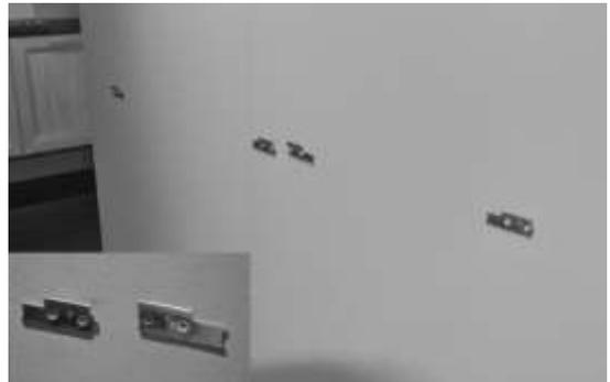
e\_ Once fixed the brackets on the wall, and checked all measures, you can proceed with the installation of the unit to the wall.
