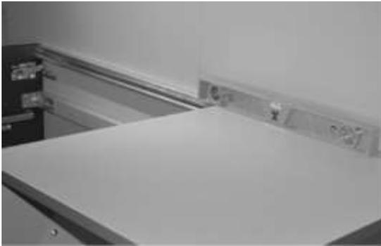
b\_ Checked the locked position of the furniture, put a level above it, as shown in the picture.
