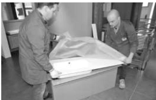
c\_ Lay the top on the cardboard box and remove the protective nylon bag making sure to always hold the element, so it will not fall or slip.
