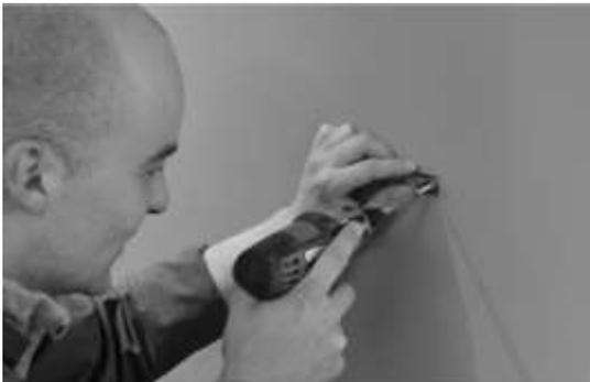
b\_ Detected points on the wall, drill the holes, insert dowels and attach the brackets.
