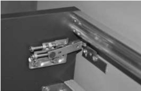
a\_ With the help of a collaborator control the exact coupling the furniture on the brackets, before letting go.
