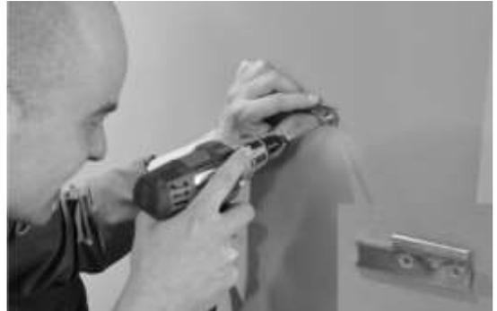
d\_ Inserted plugs in the holes, proceed to the fixing of brackets, making sure that the coupling is toward the side panel
