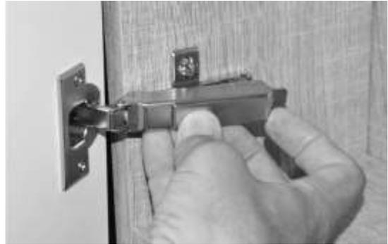
c\_ To lock the hinge, first fix the external side onto proper place, hold firmly the door.
