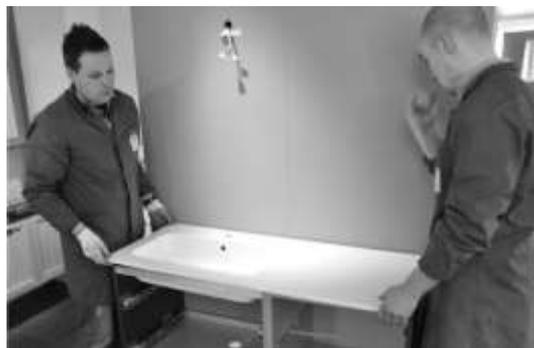
d\_ With the help of an assistant lift the top, and place it carefully above the unit.
