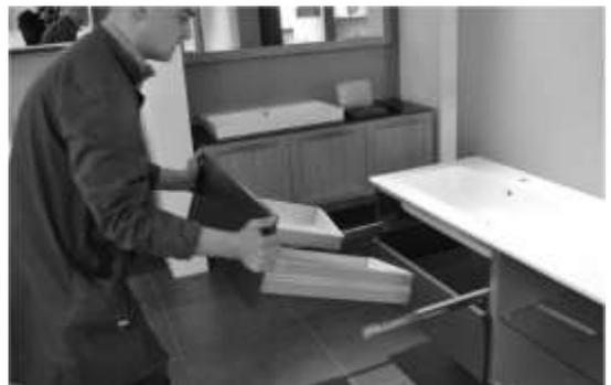
f\_ Finally, replace the drawers. This is done by extracting all of the guides, positioning the drawer above them and closing it.
